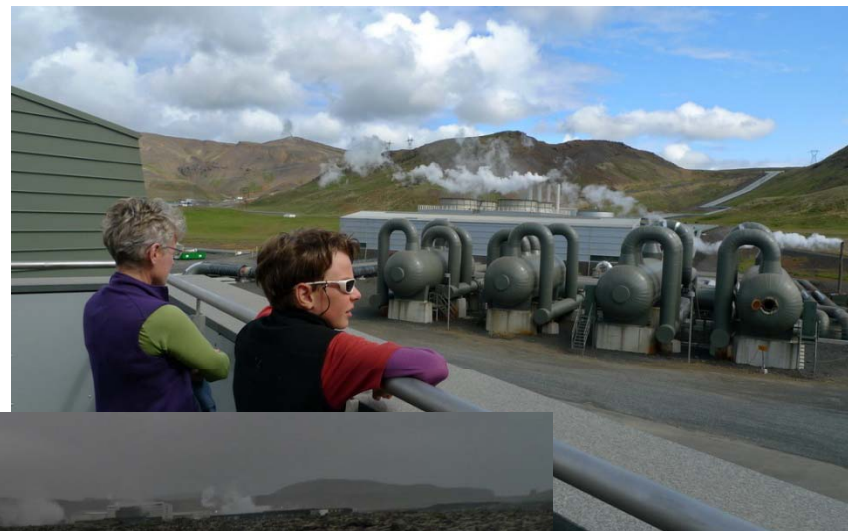
Hellisheidi geothermal power plant
